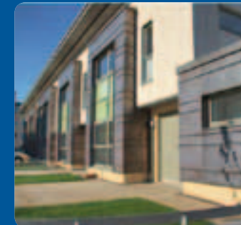
Terraced housing at Wardrop St
